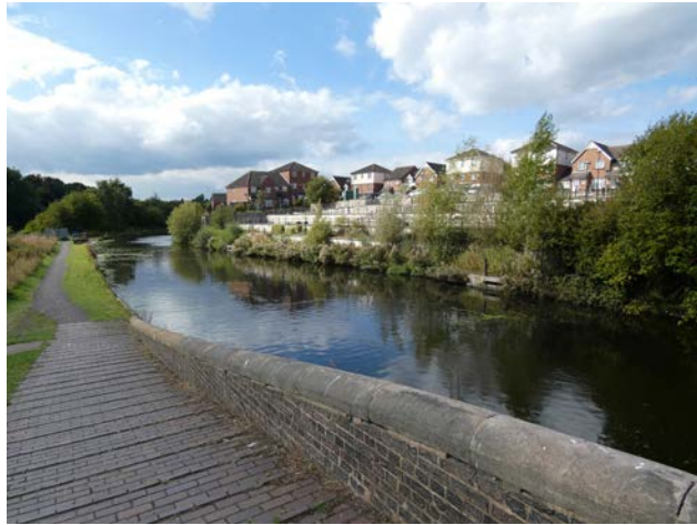
Plate 2.56 Modern concrete terracing along the Old Main Line
