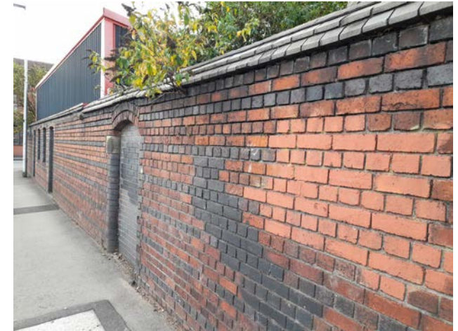
Plate 2.8 Wall to the site of the Smethwick Engine
