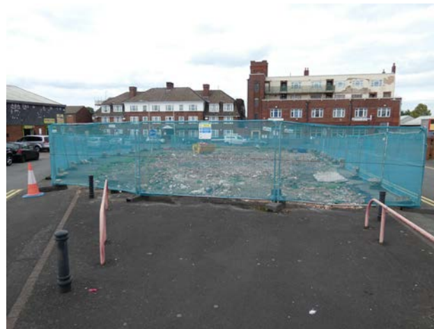
Plate 2.6 Site of the Crown and Anchor, demolished 2022
