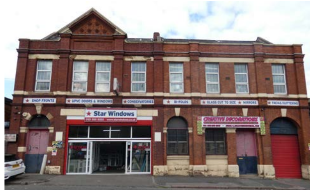
Plate 2.12 Former Post Office
