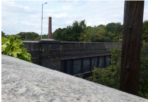
Plate 2.69 The Chimney of the pumping house over Brasshouse Lane Bridge (taken from Great Western Road)
