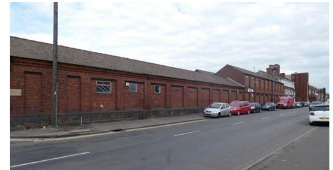
Plate 2.15 Frontage of the Enterprise Centre, former Corporation Yard
