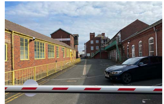
Plate 2.40 Long ranges at the Enterprise Centre site
