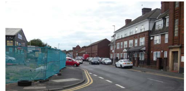
Plate 2.23 Strong frontage of the remaining buildings of the civic core
