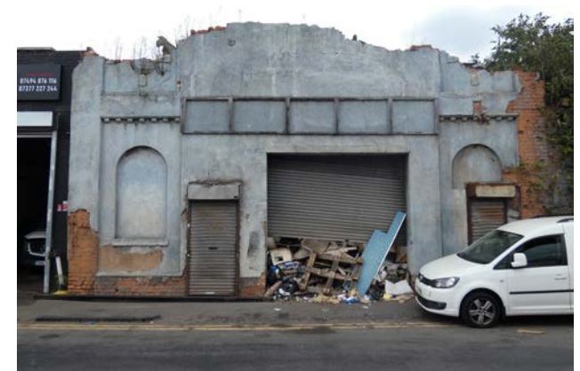
Plate 2.36 Fire damaged premises at 74 Rolfe Street
