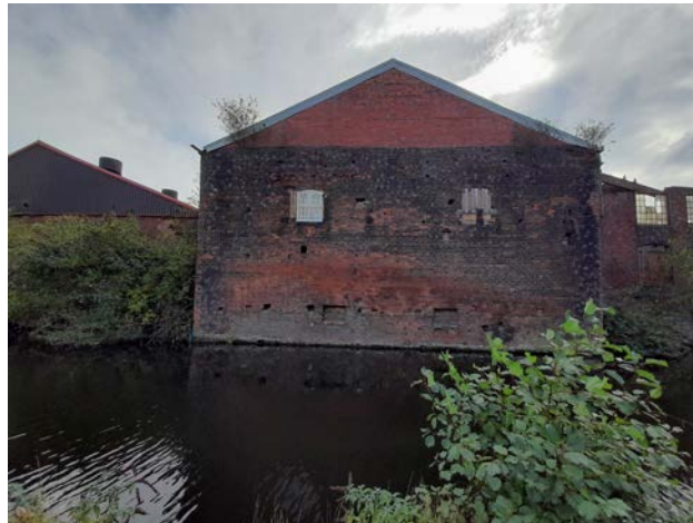
Plate 2.49 Part of 72-80 Rolfe Street fronting the Engine Arm Canal
