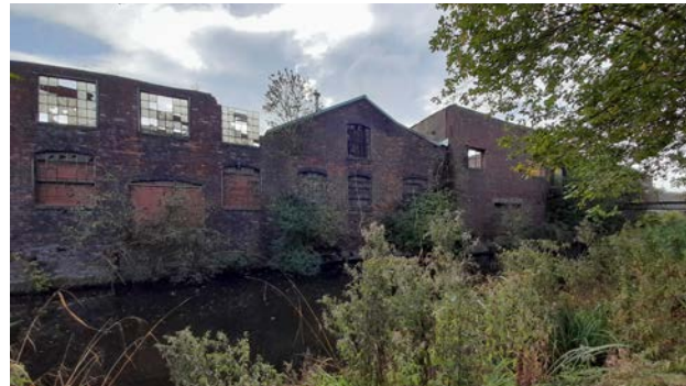
Plate 2.34 Industrial buildings fronting the Engine Arm (part of 72-80 Rolfe Street)
