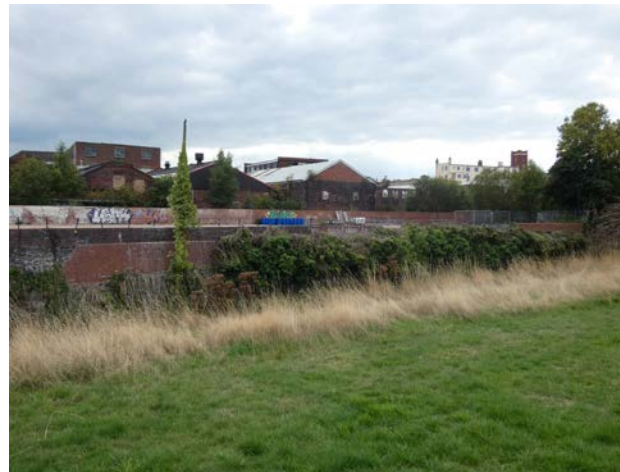
Plate 2.70 Views to the Fire Station Tower and industrial buildings from the eastern leg of the Old Main Line
